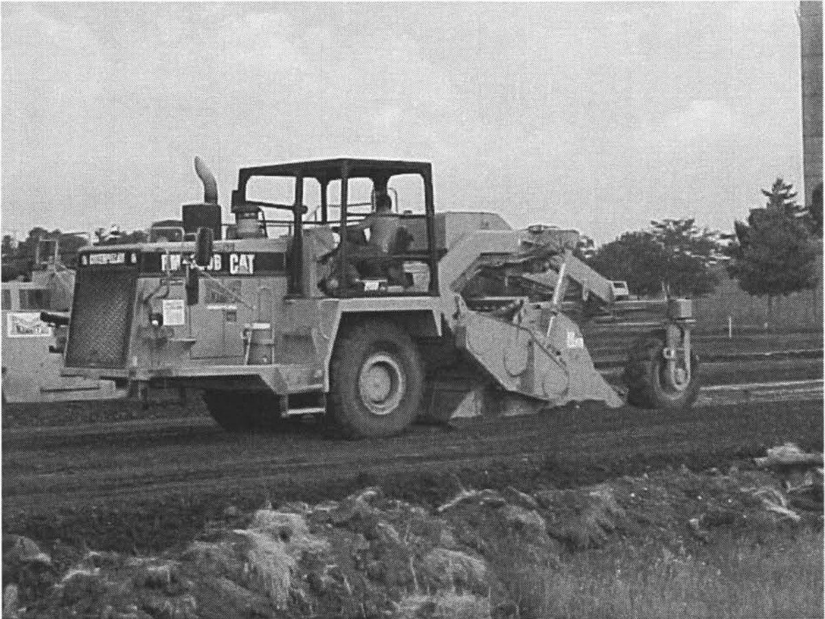
Figure 1. Typical Pulvamixer Used for On-Site Mixing
